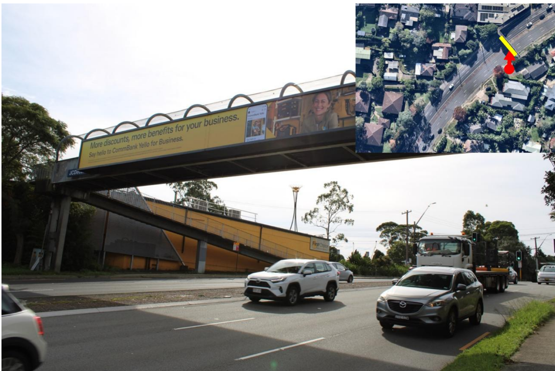
Figure 35: Looking north towards the sign from 781 Warringah Road (Source: Keylan)
