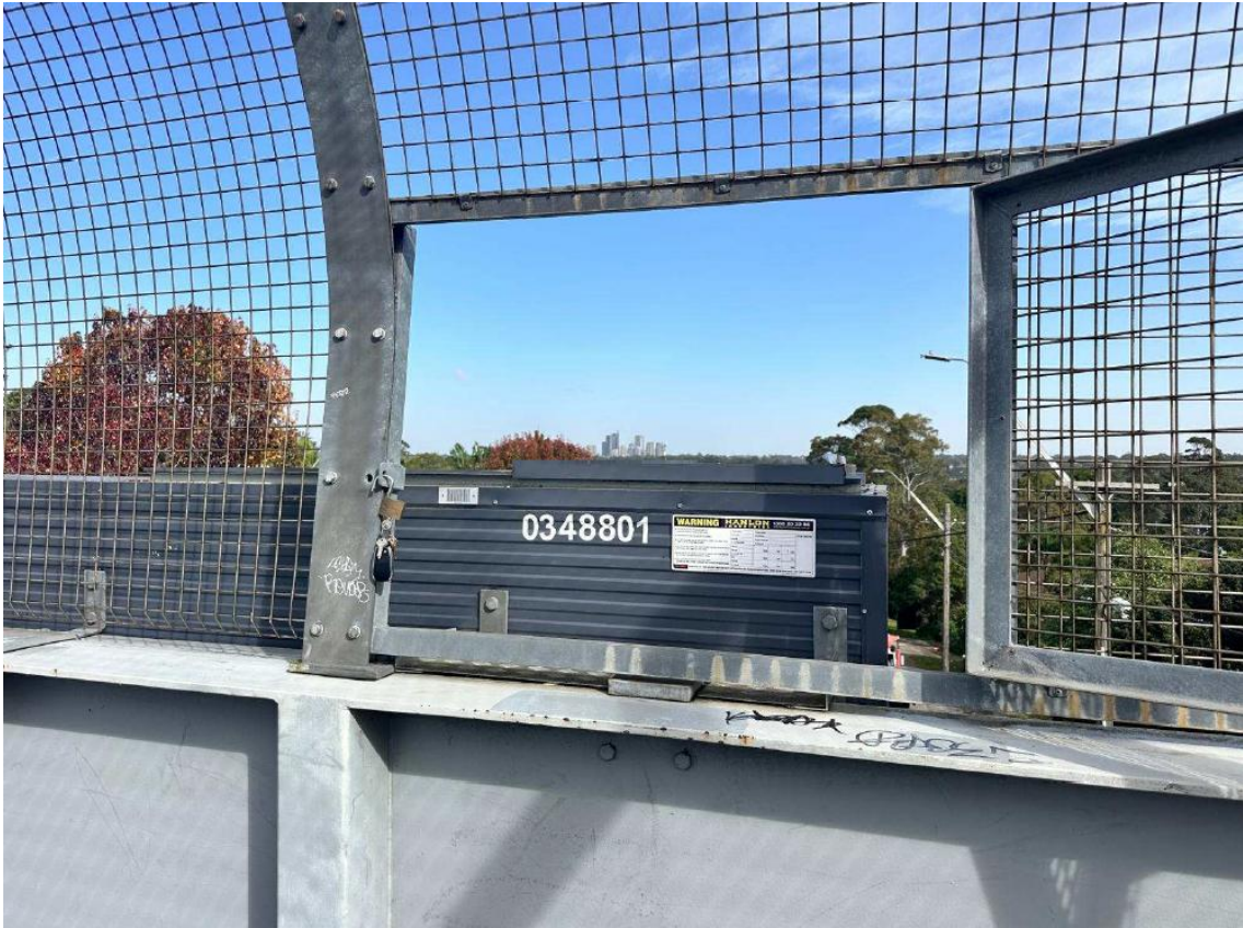
Figure 13: Access to signage (Source: Dennis Bunt Consulting Engineers)
