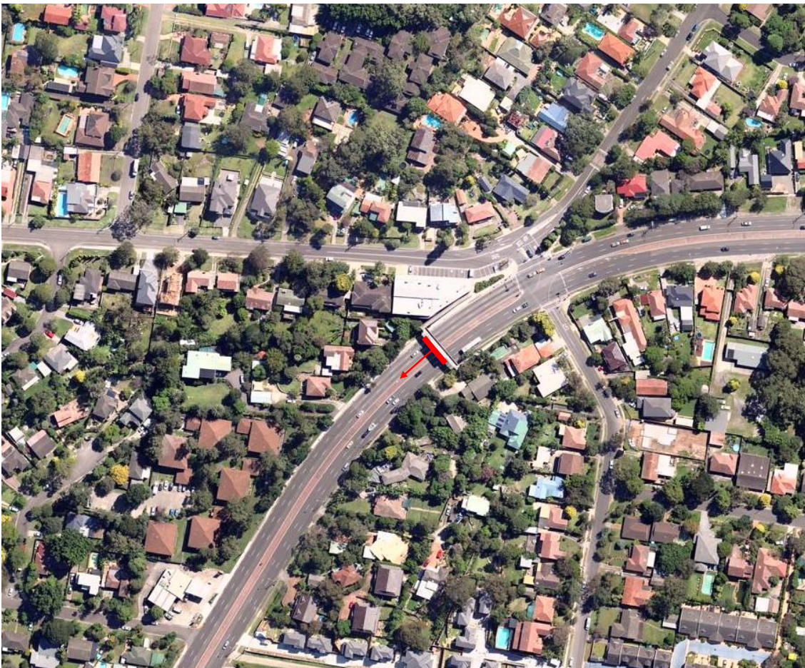
Figure 3: Aerial view of the site in 2010 (Base source: Nearmap)
