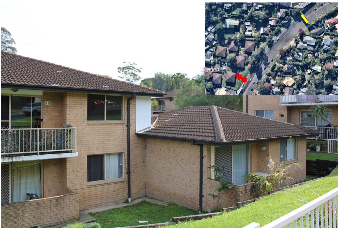
Figure 31: Looking north-west towards 9 Aldinga Place (Source: Keylan)
